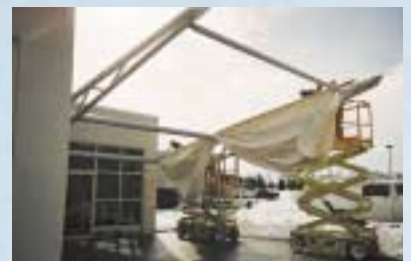
BMW display canopies at Cumberland Valley Motors, Mechanicsburg, Pennsylvania.
