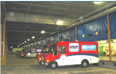
Suspended "curtains" to contain and control truck exhaust, dust, fumes, and other airborne particles.
