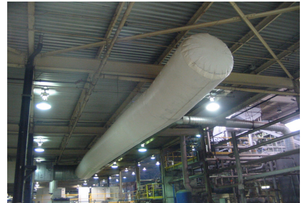
The exhaust end of a Soper's duct can be closed, open, grommited, or zippered (pictured).
